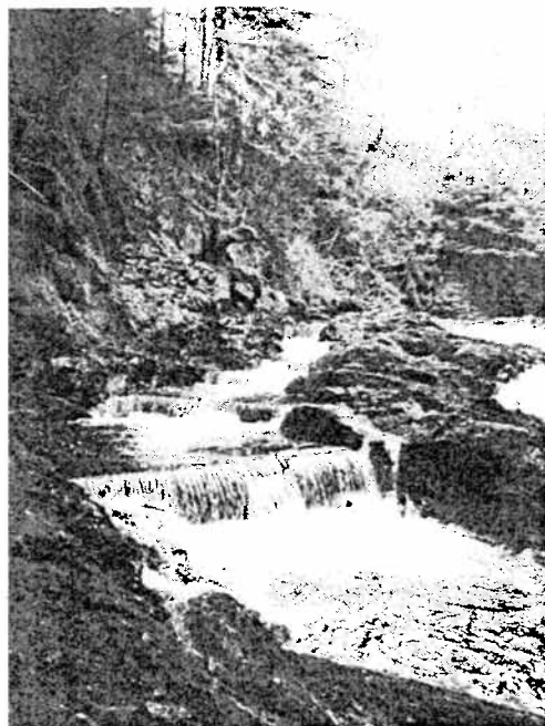
White Rock Creek blasted step-pools and weirs, Sitka RD
