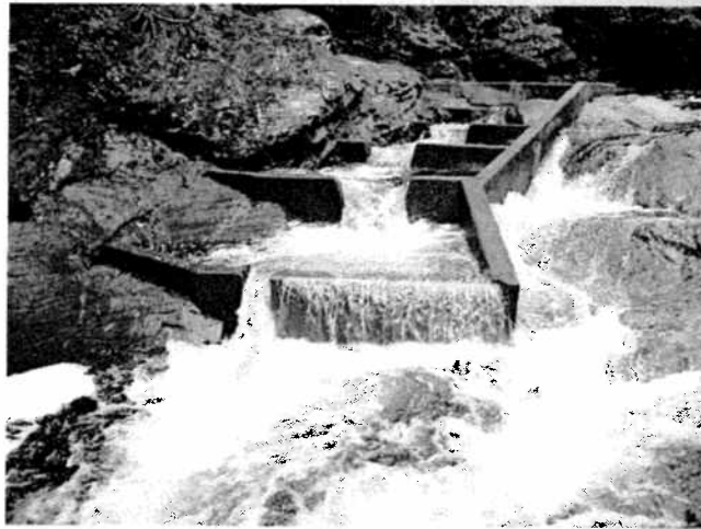
Lower Meter Bight Concrete Weirs, Wrangell RD
